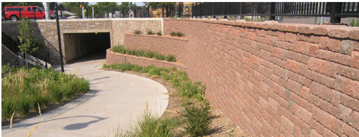
Example of Underpass Configuration for Shared Use Path
